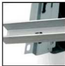
Fix footer to vertical struts using 8mm bolts provided
