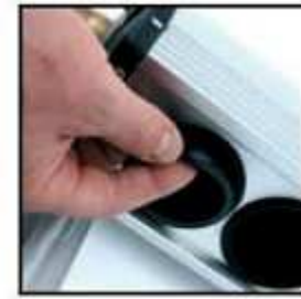
Install rubber seals into header. Lubrication recommended when installing tubes.
