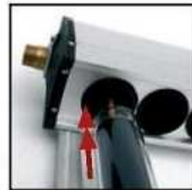
Insert glass tube through lubricated rubber into header
